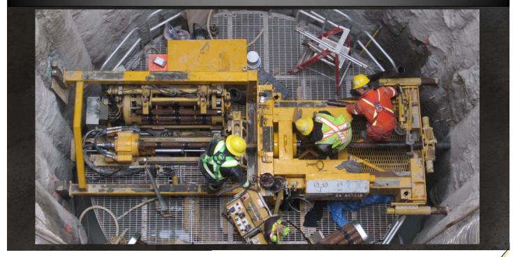
Compensation grouting, sometimes referred to as fracture grouting, involves the injection of grout to intentionally fracture the ground, creating "grout lenses" to displace the surrounding soil in order to provide controlled heave of soils and structures. It is commonly used to protect buildings by mitigating settlement caused by tunneling operations.
