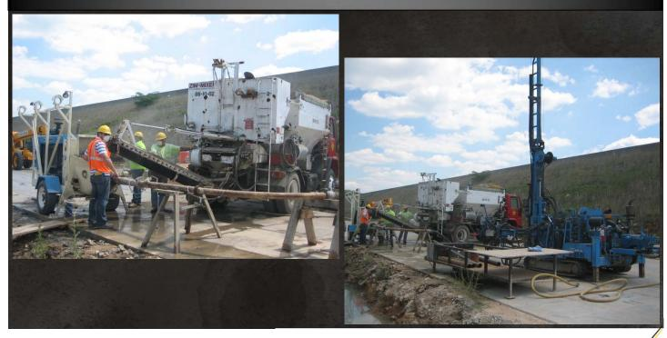
Compaction grouting is typically performed in loose or weak soils to mitigate settlements and is also used for sinkhole remediation. Compaction grouting involves the injection of a very stiff, mortar like, cementitious grout into soil to densify or compact the soil under high pressure.
