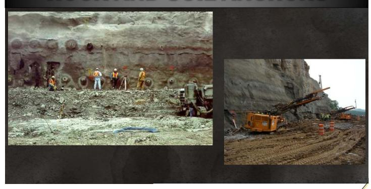
Rock and soil anchors are structural members that are used to provide temporary or permanent structural support. A rock or soil anchor consists of a tendon and an anchorage. The tendon can be one or more solid steel bars, a single hollow bar, or a bundle of high strength tensile steel strands.
