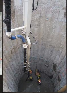
Secant Piles are constructed by drilling and concreting intersecting circular piles. Reinforcement of the piles can be achieved using either structural steel members or reinforcing steel cages.
